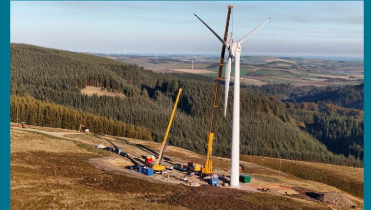
Wind turbine erection
