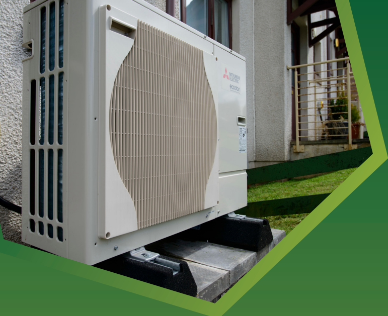
Air source heat pump, social housing, Tarbolton, South Ayrshire.
