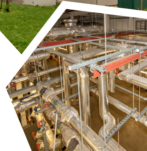
A biomass district heating system which provides 4.5 tonnes of hot water every hour to heat 700 social housing flats in Broomhill, Glasgow.
