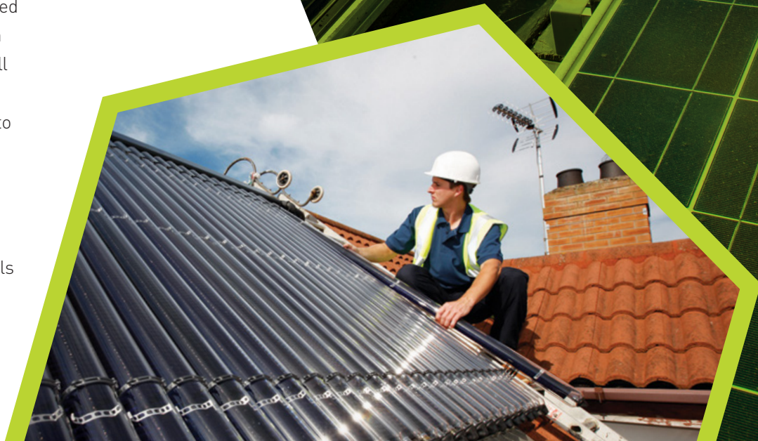
Solar thermal evacuated tubes (left) and solar PV panels (right), Castle Semple Country Park, Renfrewshire.
