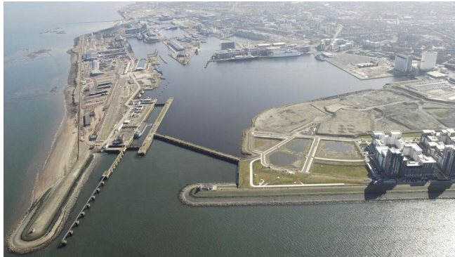
Pile Casing Marshalling – Saipem - Port of Leith
