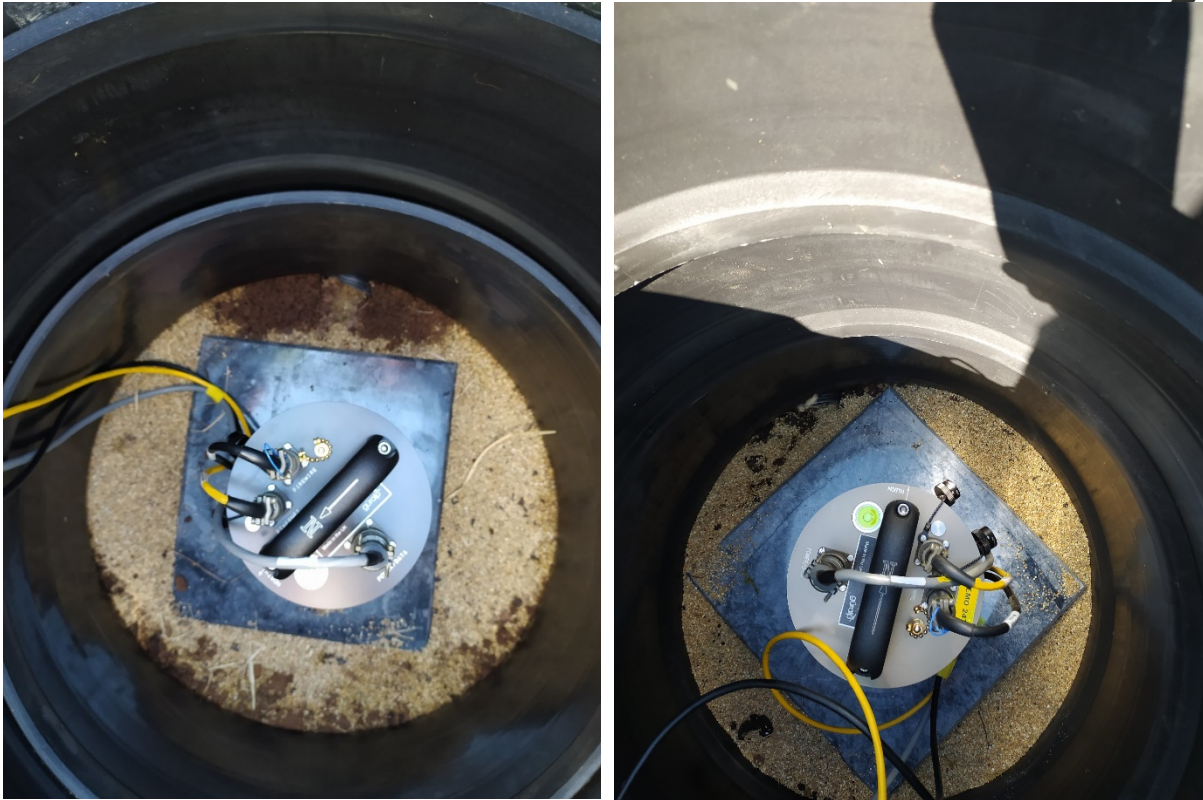
Figure 17 - Installation of the sensors at two measurement locations. Sensor resting on the slab prior to being covered by insulation.
