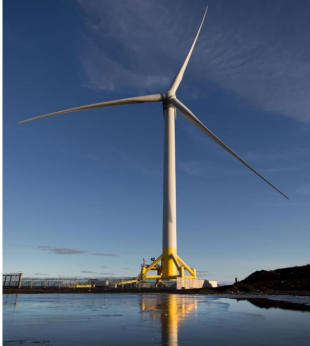
ORE Catapult 7MW Turbine Levenmouth in Fife
