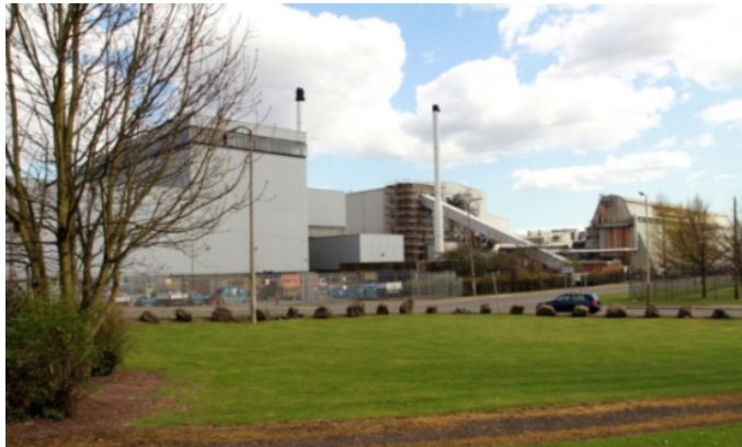
Waste to Energy plant
