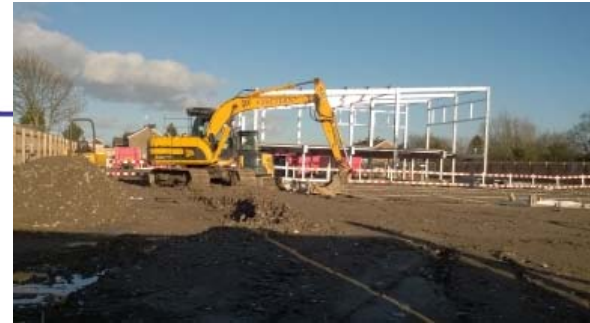
Installation of Leighton Buzzard building housed battery
