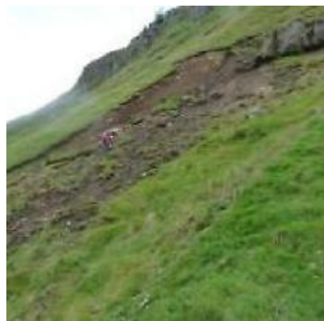
Landslip on steep ground
