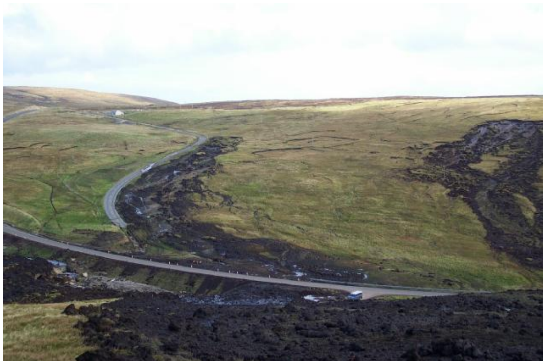
Peat slide impacting road
