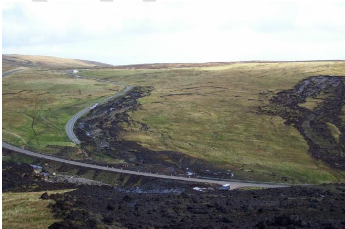
Peat slide impacting road
