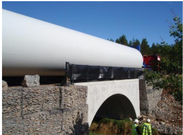
Note the bridge spans the banks of the water course to allow mammal passage under the road.
