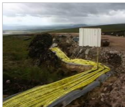
Cable trench adjacent to constructed road
