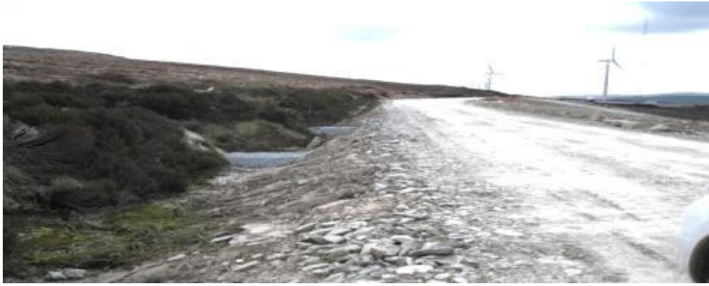
Regular, robust check dams on road sloping ditches
