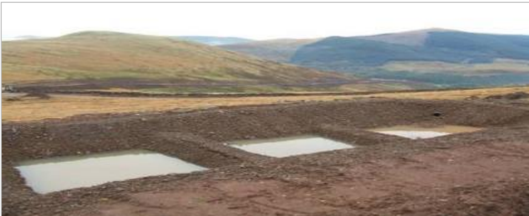
In some locations substantial 'Step' designed settlement lagoons may be required to manage large volumes of contaminated run-off.
