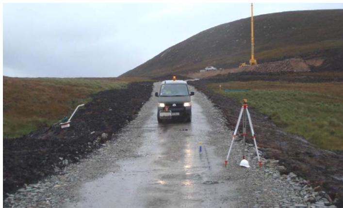
Surveying floating road structural integrity. Note that excessive material should not be placed on the side of tracks as shown on the left of this image.
