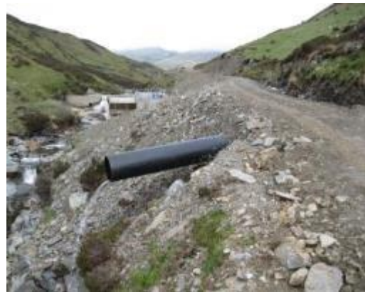
Culvert under road – shorten the pipe and apply mitigation to avoid scour of the bed.
