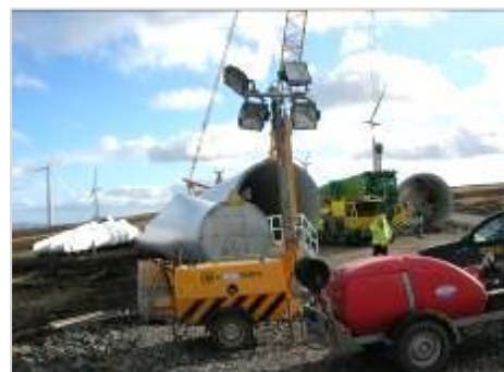
Considerable lay-down areas are required on site and should be planned for early in the process.
