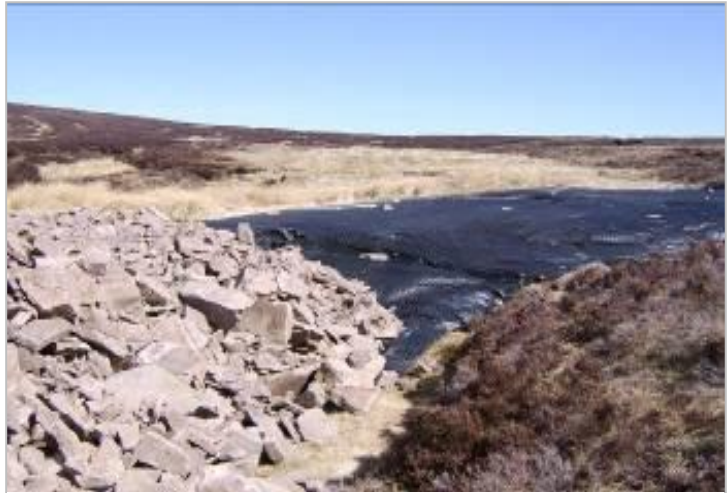
Poor floating road construction - attention to detail is required at track edges to prevent construction material spilling onto surrounding vegetation. Tipping large aggregate onto the geogrid, as shown, is unlikely to create the necessary interlock with the geo-grid.
