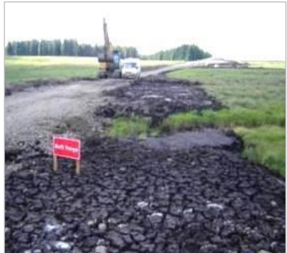
An example of poor practice. Excavated peat placed 4m from edge of access track. Note that no peat turves have been re-used. This peat is likely to dry out and provides no ecological benefit.
