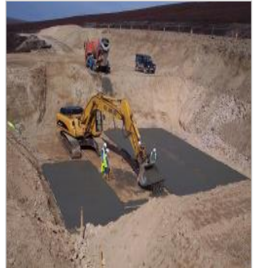
Preparation of turbine foundations
