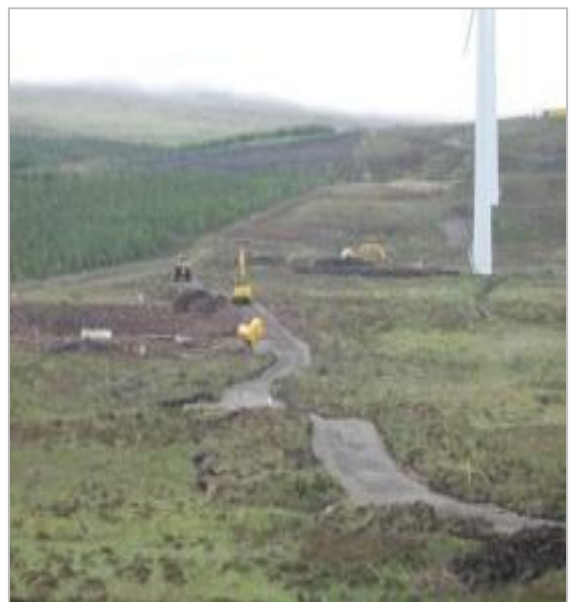
An example of good practice. Track edges have been reinstated with whole turves and tied into the surrounding landscape.
