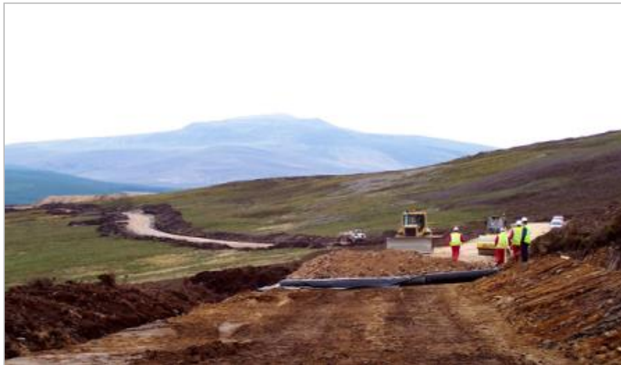
Construction of a cut road
