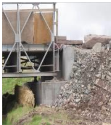
Temporary construction phase bridge and bank habitat. Steep sides of loose material could be washed off in a storm event. Use of splash boards on bridges can prevent contamination of watercourses.
