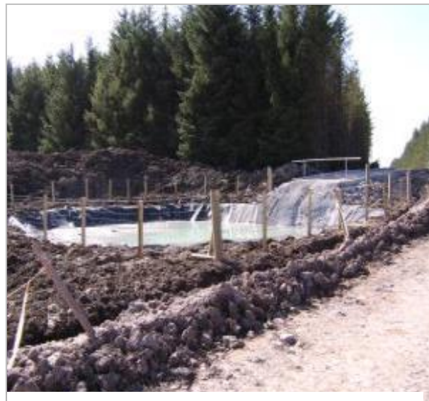
A well designed and located cement wash out bay can prevent bad practice elsewhere on site. A ticketing system to ensure it is used by all drivers has been shown to be useful.
