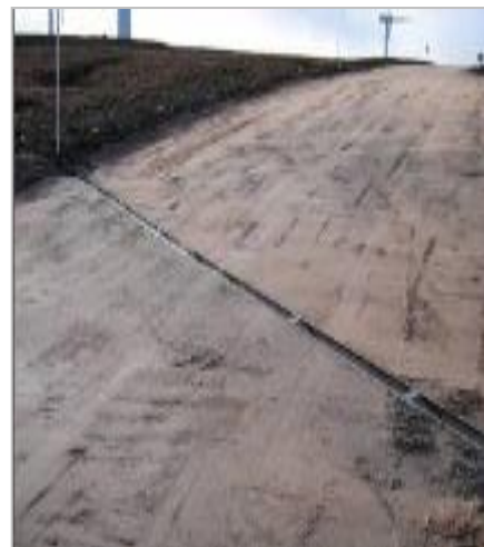
Cross-drain on access track. Good practice would cover the drain with a screen to prevent debris entering.
