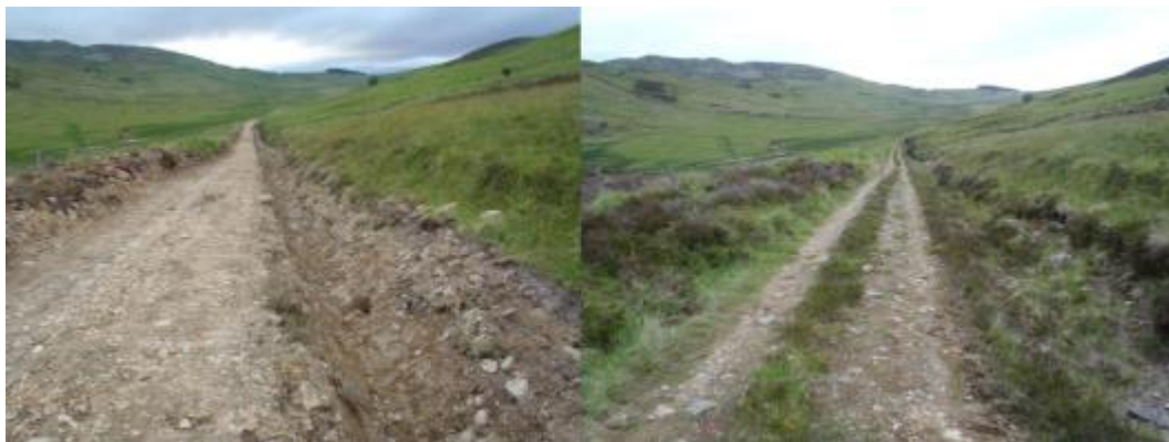
Effective track reinstatement
